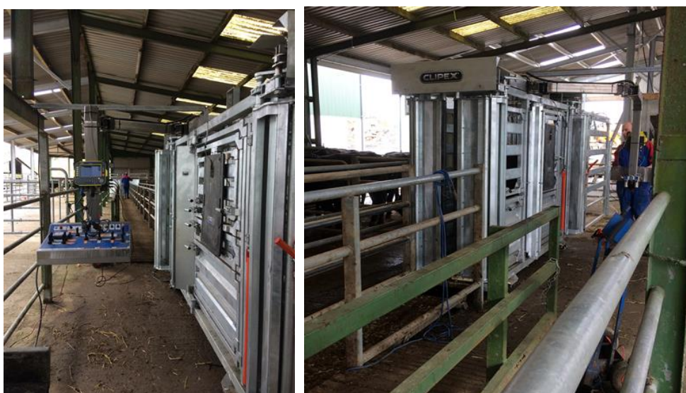
New Clipex weighing facility
