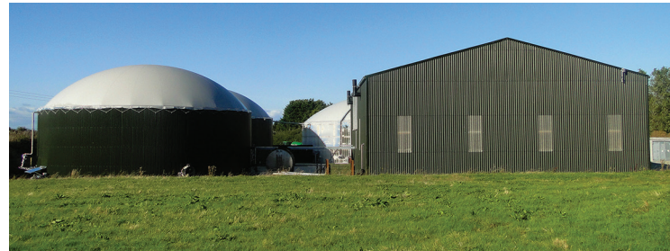
Figure 5. Anaerobic Digestion Plant supported by REFIT 3, Shanagolden, Co. Limerick (Source: McDonnell Farms Biogas Ltd)
