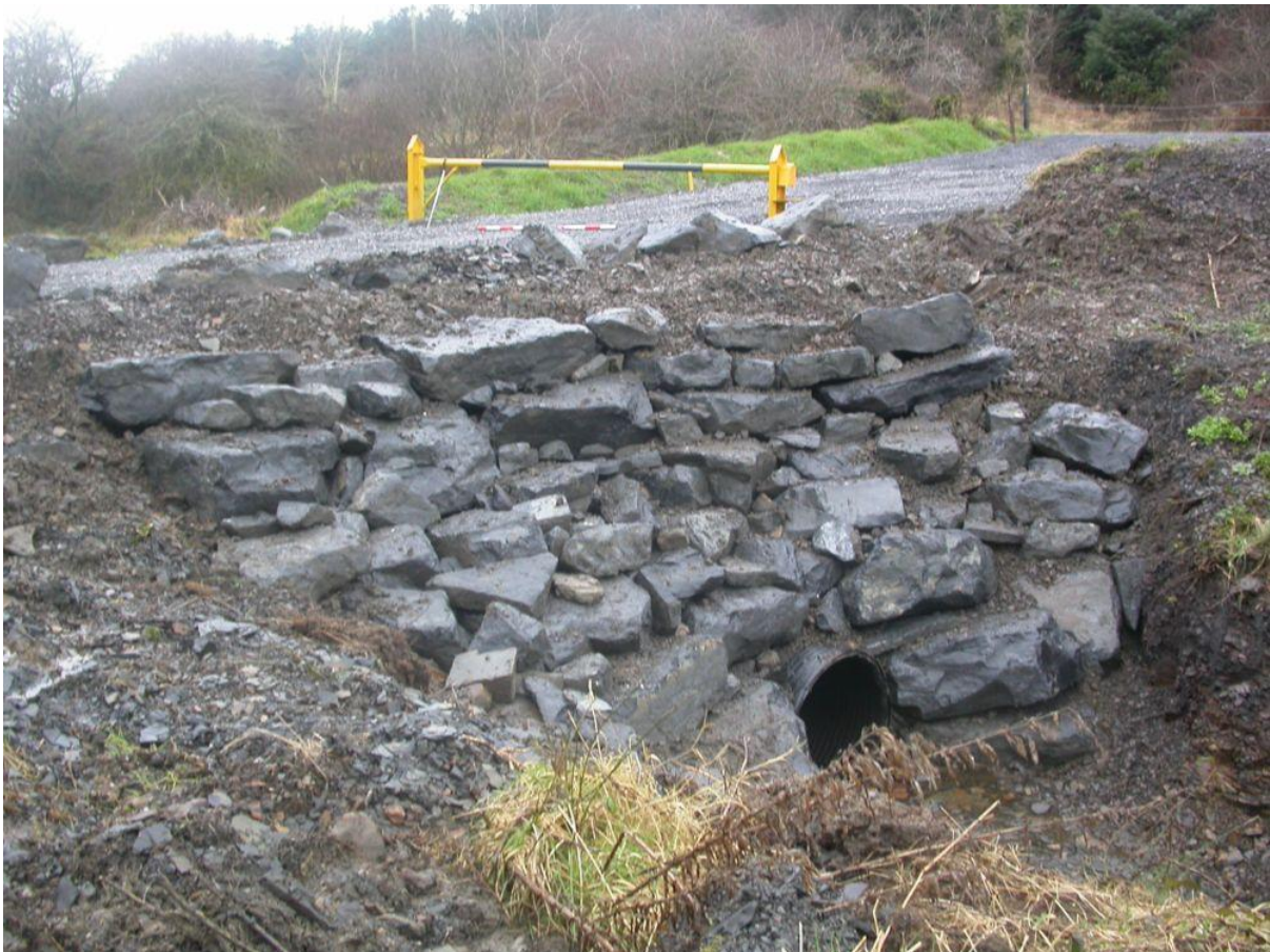
Picture 6: Drainage under a forest road entrance.
