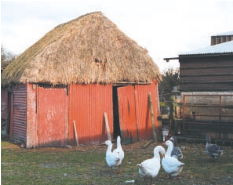
Thatched hen house. (left) Thatched hen house with corrugated-iron and timber board cladding, built c.1950. Near Ballinagar, Co. Offaly
