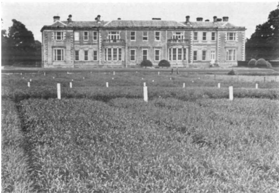
Plate 3— Headquarters of Plant Sciences and Crop Husbandry Division of the Agricultural Institute at Oakpark, Carlow.
