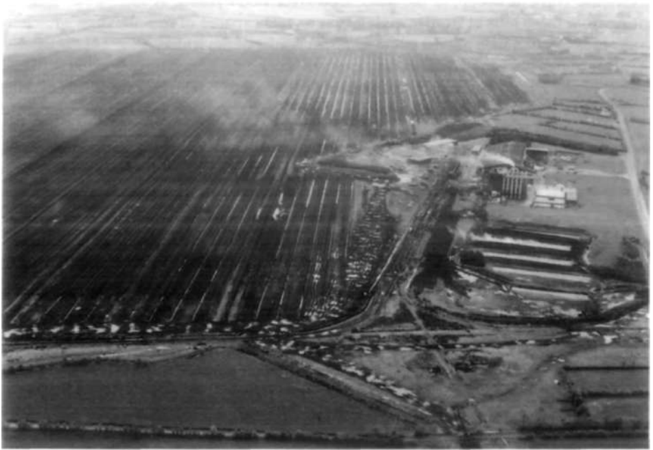
Photo 4.7. Briquette factory on lowland peat (Boora Complex), Littleton.
