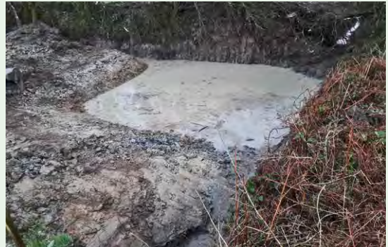
Figure 6. A settlement pond installed at a confluence of land drains to prevent sediment run-off to the River Allow (source Michael Morrissey IRD Duhallow Farming for Blue Dot Catchments EIP Project March 2021).
