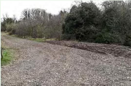
Figure 4. Farm roadway cambered with a mound installed to prevent nutrient and sediment run-off to the River Allow (source Michael Morrissey IRD Duhallow Farming for Blue Dot Catchments EIP Project March 2021).
