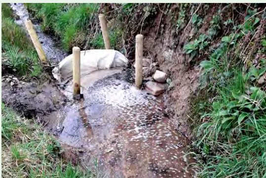
Figure 1. A bespoke silt trap installed in a fast flowing eroding land drain to prevent silt run-off to the River Allow (source Michael Morrissey IRD Duhallow Farming for Blue Dot Catchments EIP Project March 2021).
