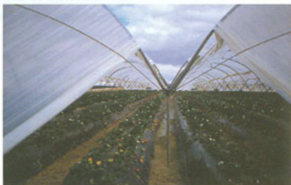
Spanish tunnel made of lightweight steel
