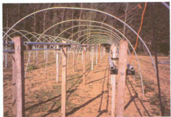
Steel and wood combination support system
