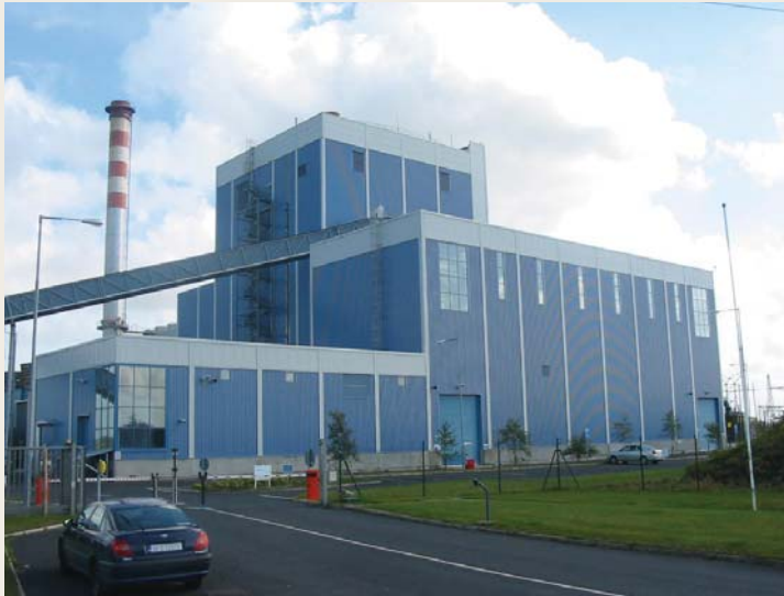
This generating station at Edenderry is well suited to the burning of biomass co-fired with peat; payment policy changes and research support will be needed for a smooth transition.
