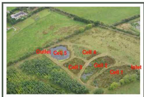
Figure 1 - Aerial view of a five year old surface flow integrated constructed wetland in the Anne Valley, Co. Waterford, Ireland (Carty et al., 2008).
