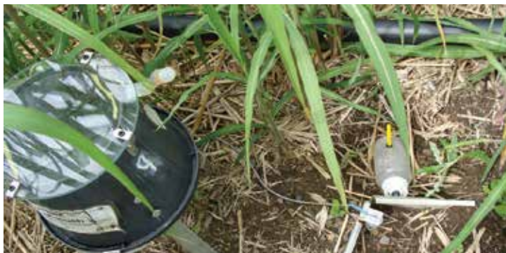
Installation of V-notch weir, and overland flow indicator (plus protective bucket with solar panel for power). Note the brewer's waste irrigation pipe in the top right hand corner of the picture.
