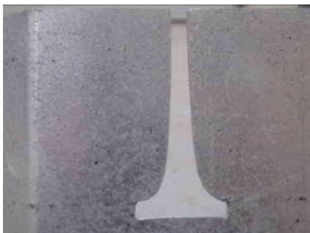
Sutro weir (left). Sutro weir installed at Hillsborough (right)
