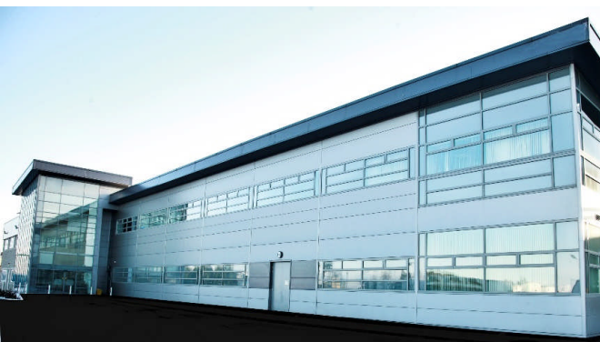
PLANT 1 NAAS, IRELAND
