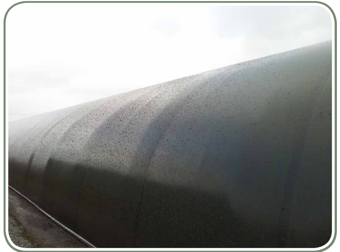
14. Compost dust on a growing tunnel roof after emptying reinforces the importance of effective end of crop steam cook-out
