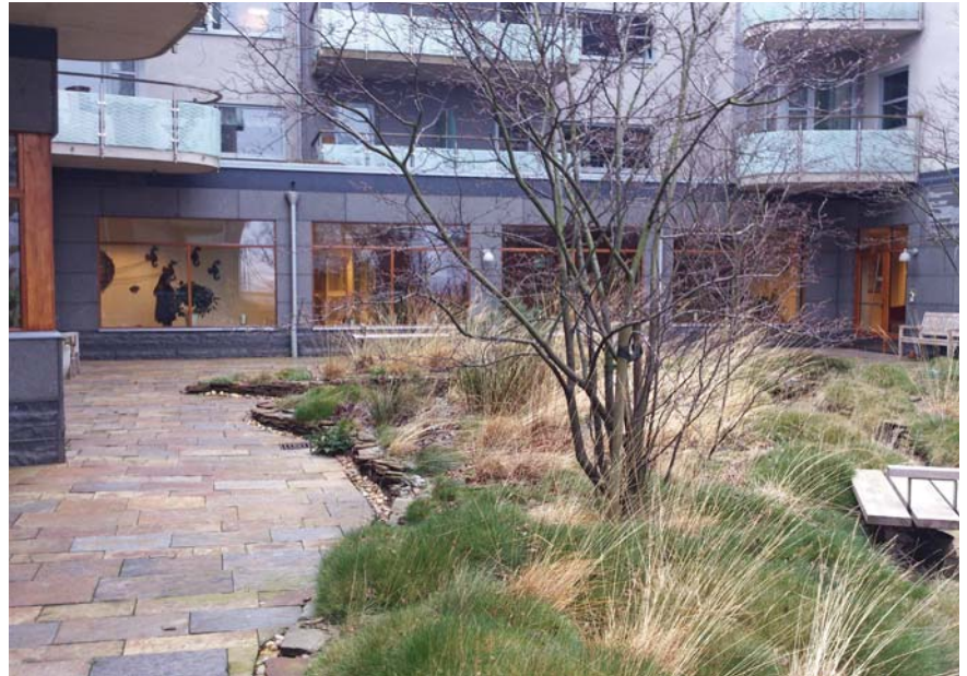
Award-winning apartments in Malmö, Sweden, use rain gardens in courtyards to drain water from hard surfaces.
