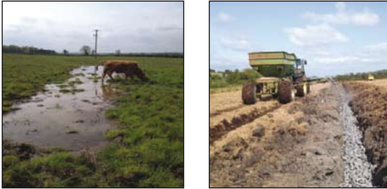
Figure 1. Surface waterlogging on poorly-drained grassland (left) and drainage installation (right).
