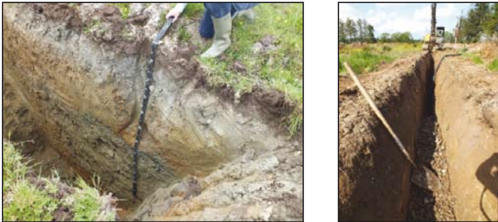
Figure 2. Test pit excavation (left) and drainage trench excavation (right).
