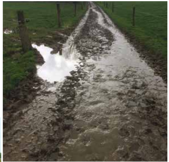
Water trapped on the roadway lodges at low points. Cattle are following tracks due to a less than perfect surface.
