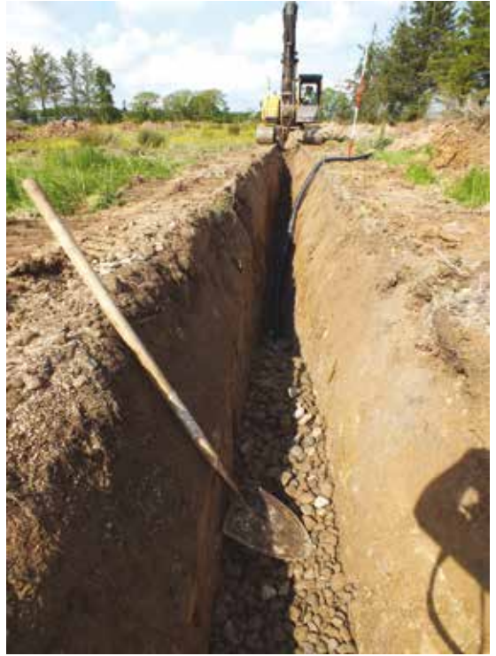
Drainage trench excavation
