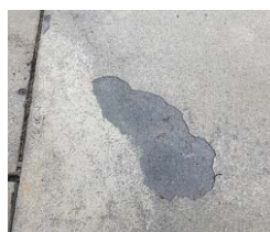
Flaking and fading on sandstone.
