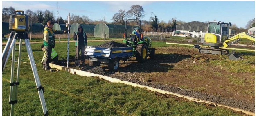
First-year students from our Level 7 degree programme can be seen here checking levels and falls while constructing a capillary bed on the campus in Teagasc Ashtown. This is part of the landscape construction module which is in conjunction with Waterford Institute of Technology.
