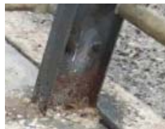
Stanchion showing corrosion. Painting the base of stanchions and cubicles will prolong their life.
