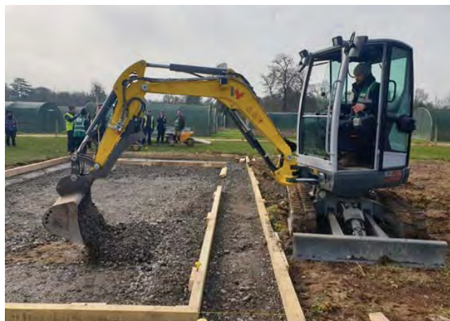
First-year students from our Level 7 degree programme can be seen here checking levels and falls while constructing a capillary bed on the campus in Teagasc Ashtown. This is part of the landscape construction module which is in conjunction with Waterford Institute of Technology.
