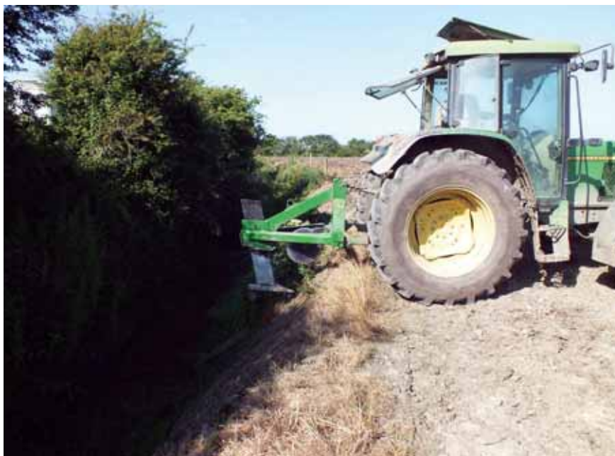
Installing mole drains.
