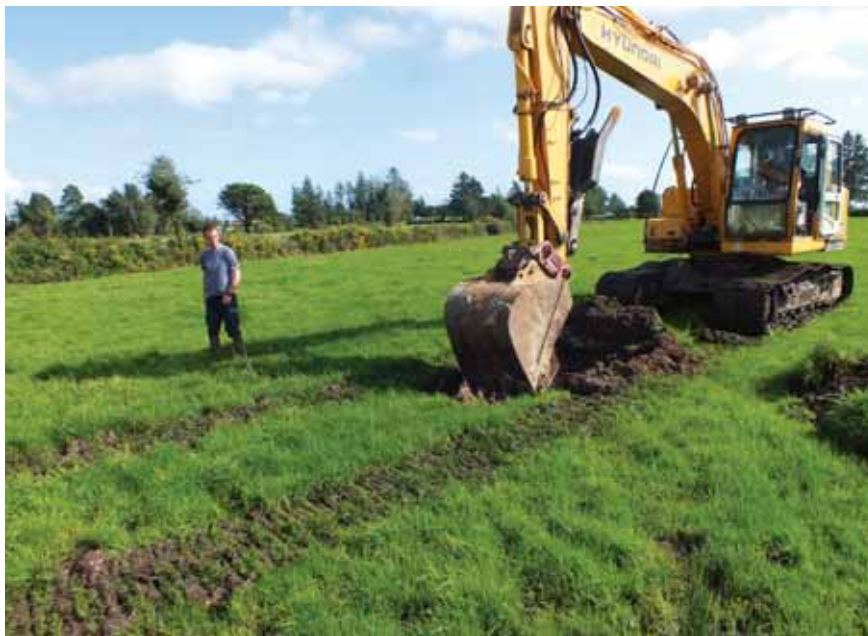
Excavating a test pit.
