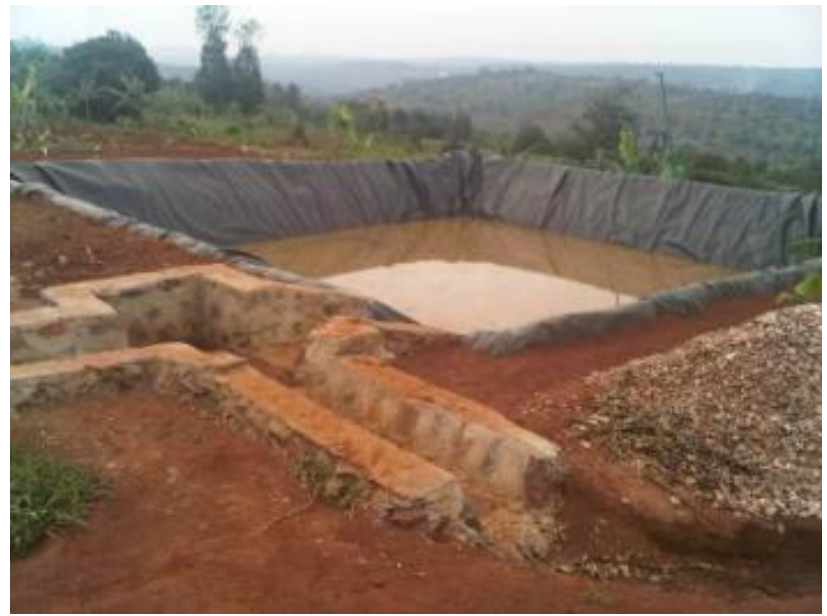
Road run-off water harvesting ponds, Burundi
