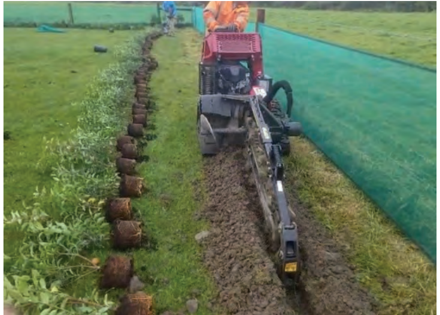
A trencher positioned 1.2m away from boundary fencing planting 3 Lt potted prunus with a wind-breaker attached to the boundary fence.
