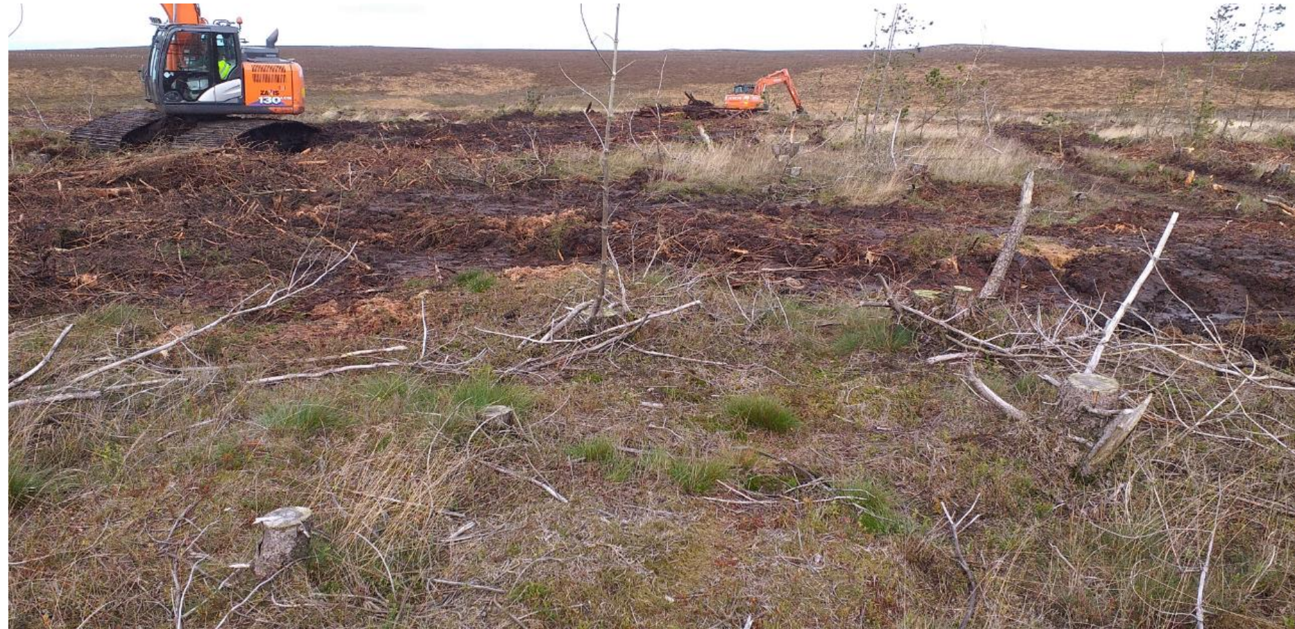
40 year old mole drains, trenched, dammed & banded.
