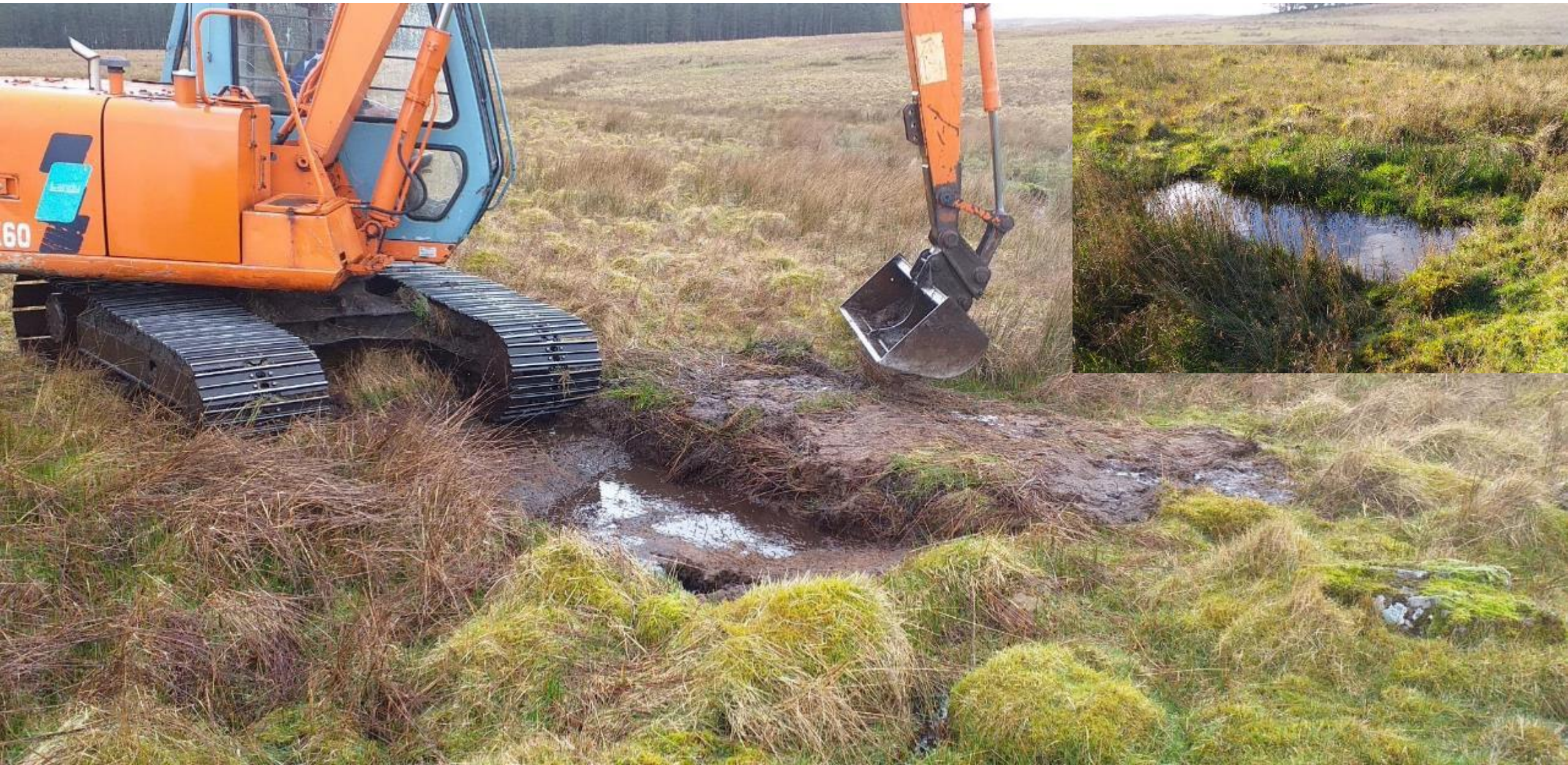
Creeve Park – Feb 2021 Provision of multiple water sources - mineral soil scrapes & moorland dams
