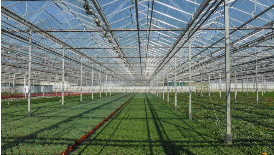
Westland Greenhouse, Wateringen, The Netherlands (Source: Flickr/ Jeroen van Luin, Creative Commons)
