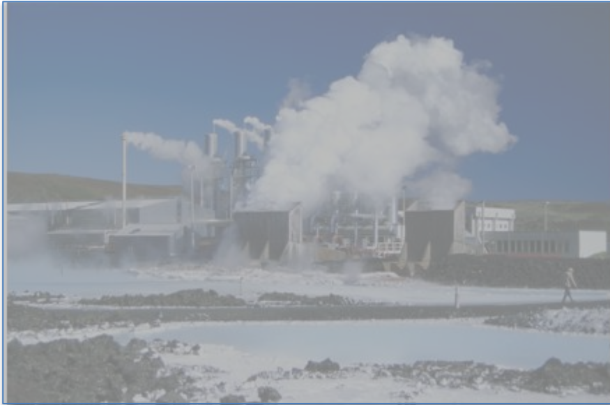
Svartsengi geothermal power station, Iceland
