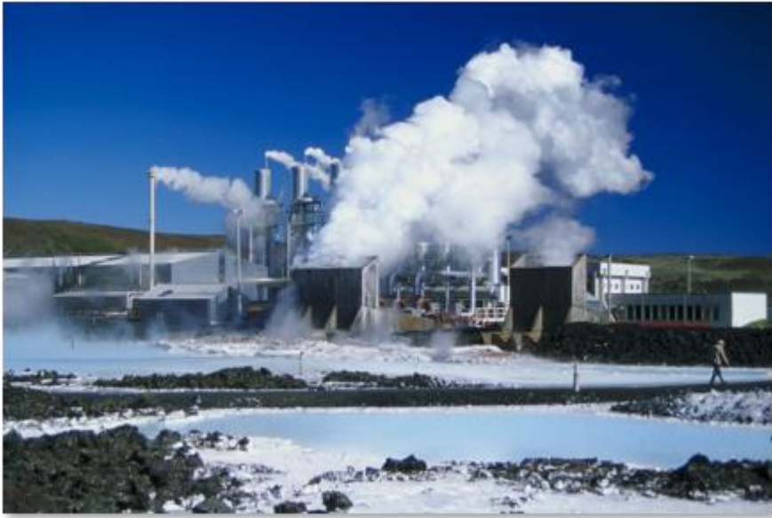
Svartsengi geothermal power station, Iceland
