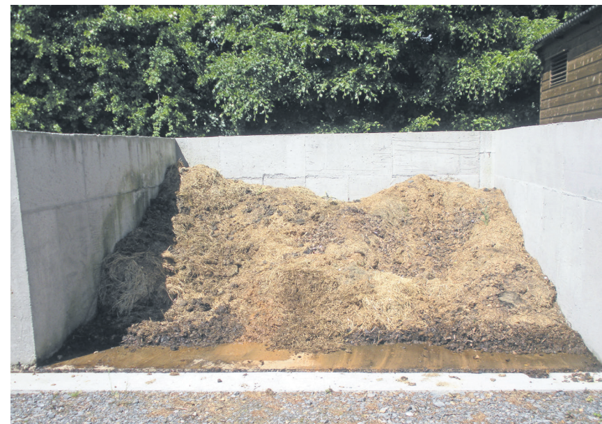
Manure pit with channel to divert effluent to underground tank \ Wendy Conlon
