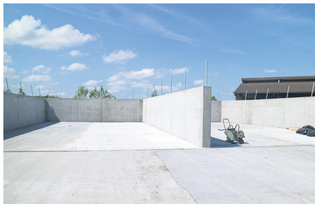
Sean's new silage pits were completed just in time for silage 2018.
