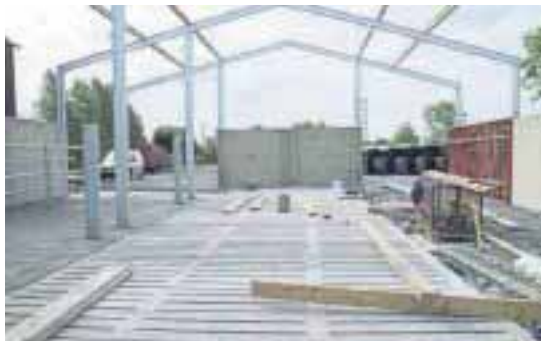
Nigel O’Kane’s shed during construction.
