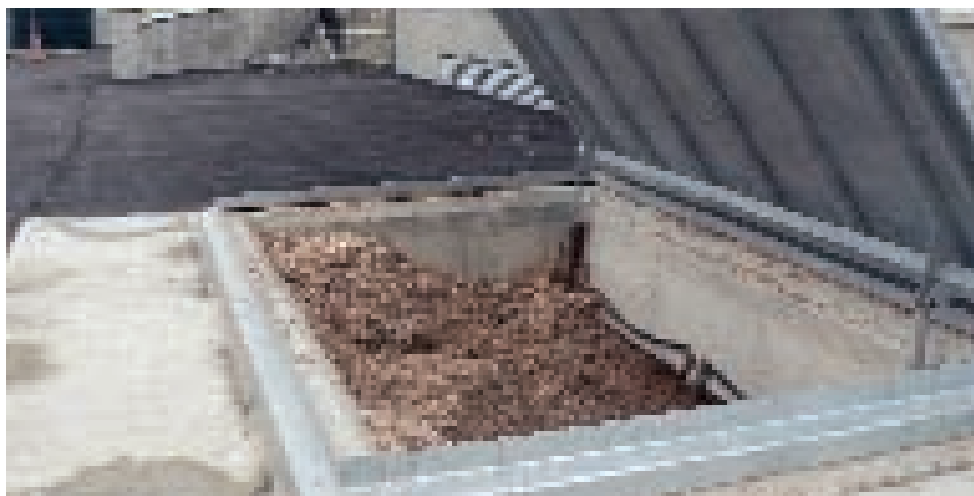
Wood chip bunker
