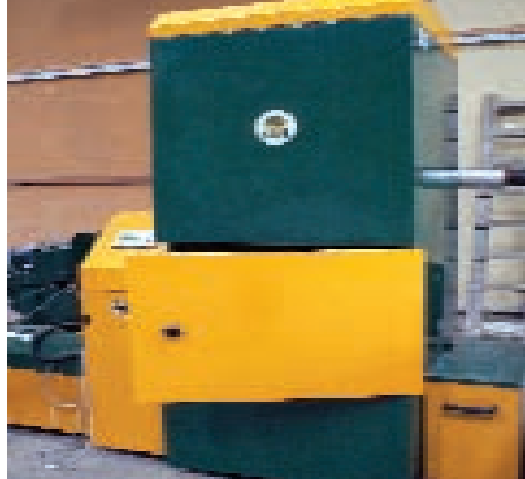
Wood chip central heating boiler
