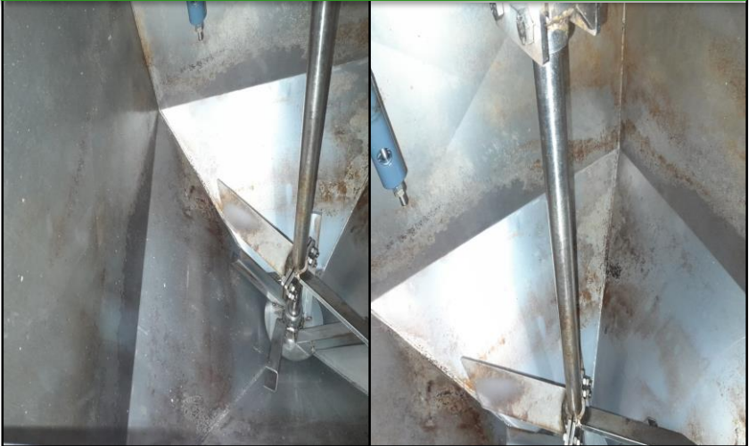
Mixing tank scrubbed and power washed
