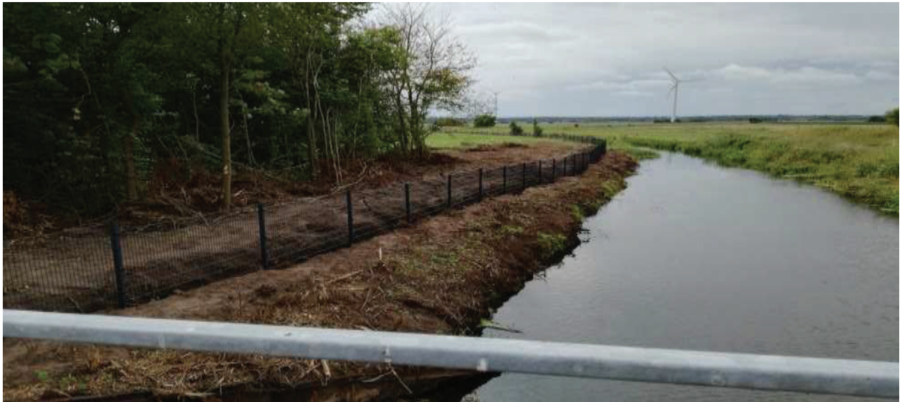
Fig. 3. Border Fence along border between Germany and Denmark.
