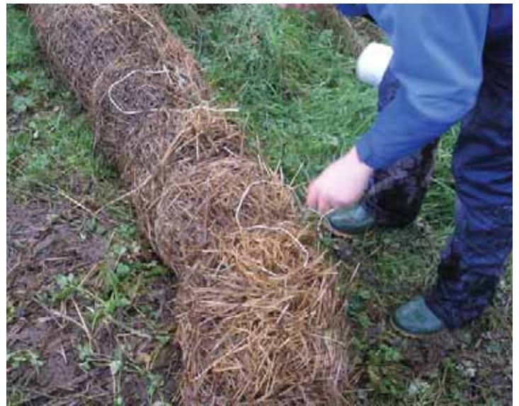
Barley bale construction.
