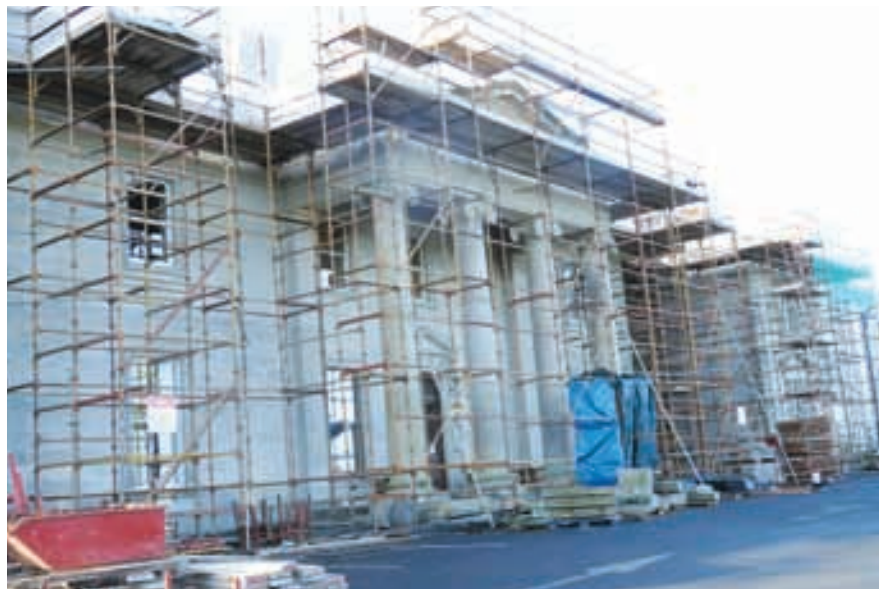
Roof repairs underway at Oak Park House, Carlow.
