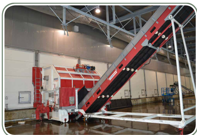
6 & 7. Clean equipment, ready for emptying tunnels
