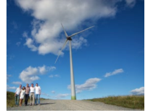
Onshore Wind Energy
