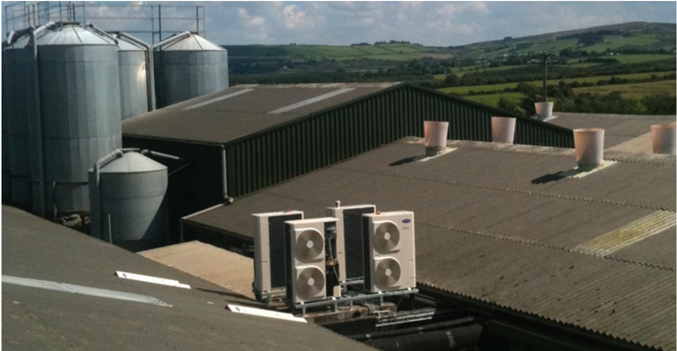
The size of the heat pump should be matched to a building's heating requirements.
